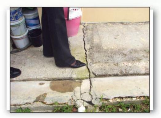
Additionally, I observed that there was an absence of a proper drainage system within the property and the back of the house was water logged even though it had not rained for several days. It would appear that the lack of proper drainage compromised the integrity of the structure, which undoubtedly would prove unable to withstand storm and earthquake activity. Furthermore, this structure contained several other noticeable defects, some of which are listed hereunder:
